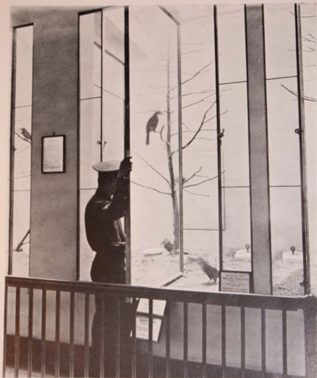
DETAIL OF PIVOTED GLASS CAGE FRONT
